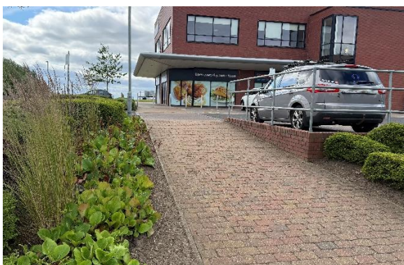
Accessible pedestrian route incorporating a step-free ramp with appropriate surfacing and clear access to shop entrance.
