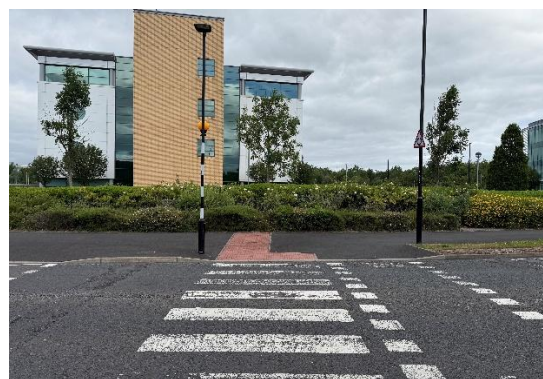
Defined pedestrian crossing with tactile paving and clear markings to support safe and inclusive street crossing.
