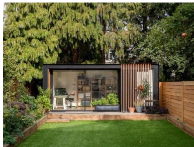
Contemporary outbuilding combining timber, glass and steel.
