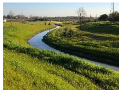
Swales conveying and attenuating surface water across the site.
