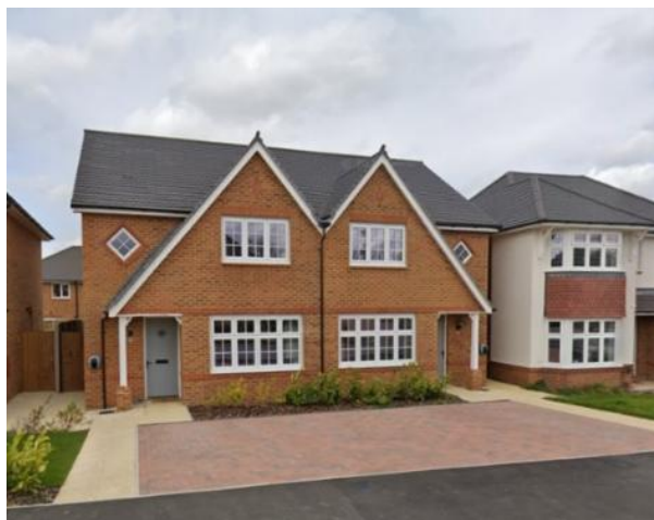
Block-paved parking with a separate footpath and soft landscaping.
