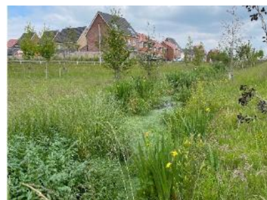
Detention ponds providing surface water storage and habitat.
