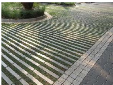
Permeable surfaces allowing water to drain naturally.
