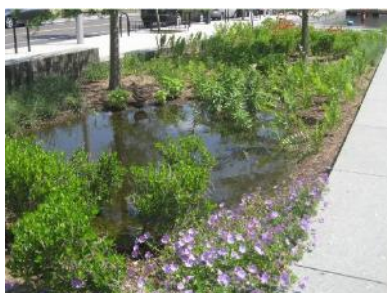
Rain gardens capturing and filtering surface water runoff.
