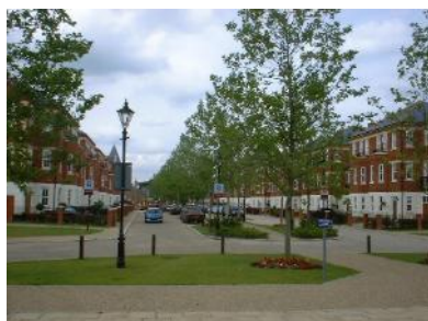
Street trees contributing to drainage and urban greening.
