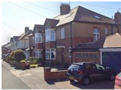
Consistent hipped roof form across the street, Tynemouth.
