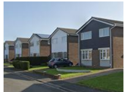
Consistent gable roof form across the street, Killingworth.
