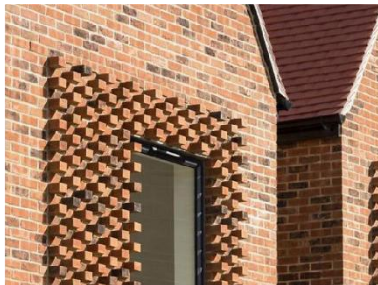
Feature brickwork patterns.
