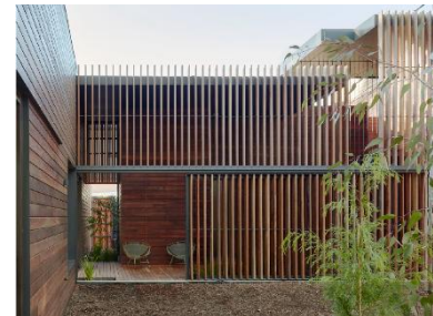
Louvres and screens.
