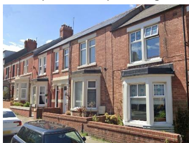
Single-height bay windows, Wallsend.
