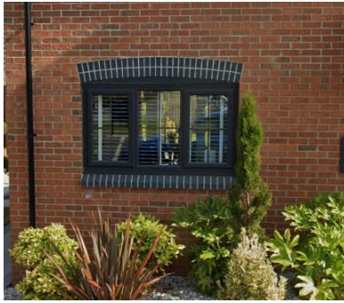
Brick header and arch detailing.
