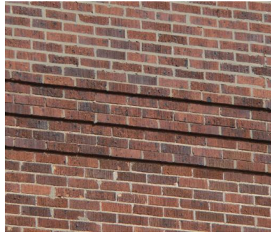
Decorative brick courses and detailing.
