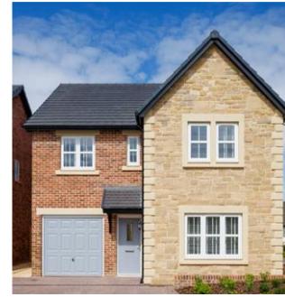
Stone cills, headers and quoins.
