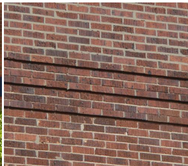
Decorative brick courses and detailing.
