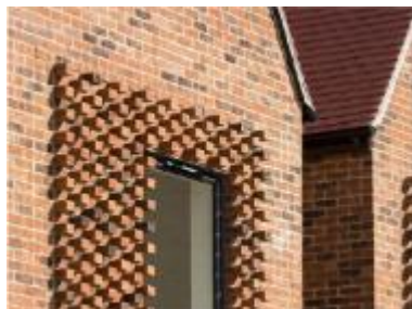
Feature brickwork patterns .
