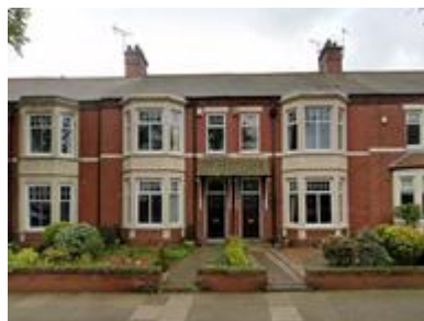
Uniform pitched slate roofs defining local character, North Shields.
