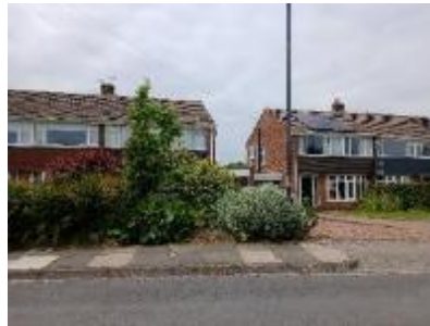
Horizontally proportioned windows, Wideopen.
