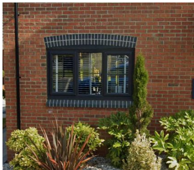
Brick header and arch detailing.
