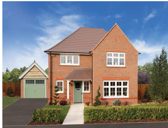
Detached garage set behind the building line.
