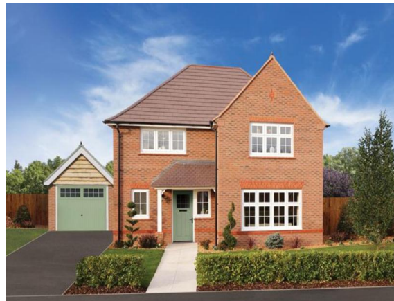
Detached garage set behind the building line.
