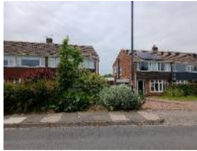
Horizontally proportioned windows, Wideopen.
