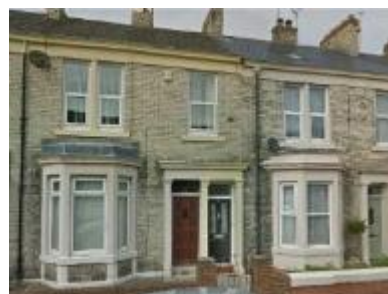
Buff brick reflecting local material palette, North Shields.
