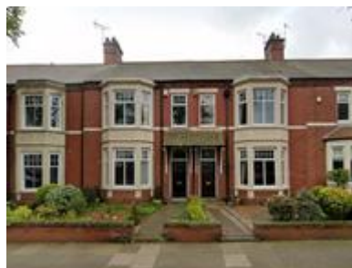
Uniform pitched slate roofs defining local character, North Shields.
