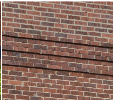
Decorative brick courses and detailing.
