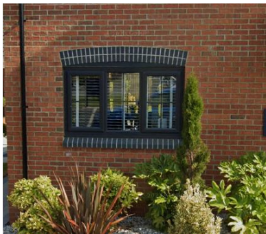
Brick header and arch detailing.
