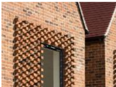
Feature brickwork patterns .
